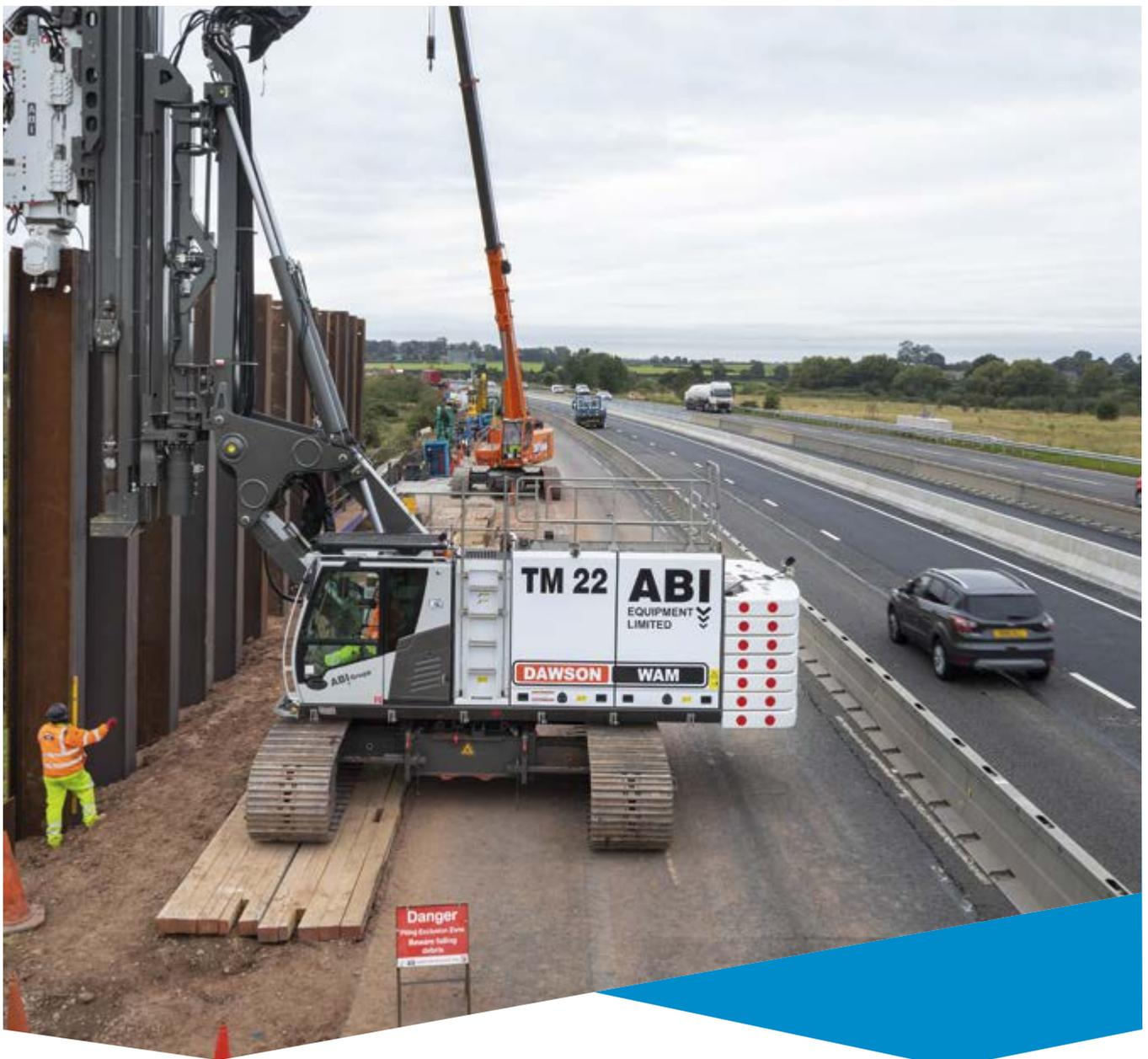
**Picture:** The last sheet pile to be installed on the project.
