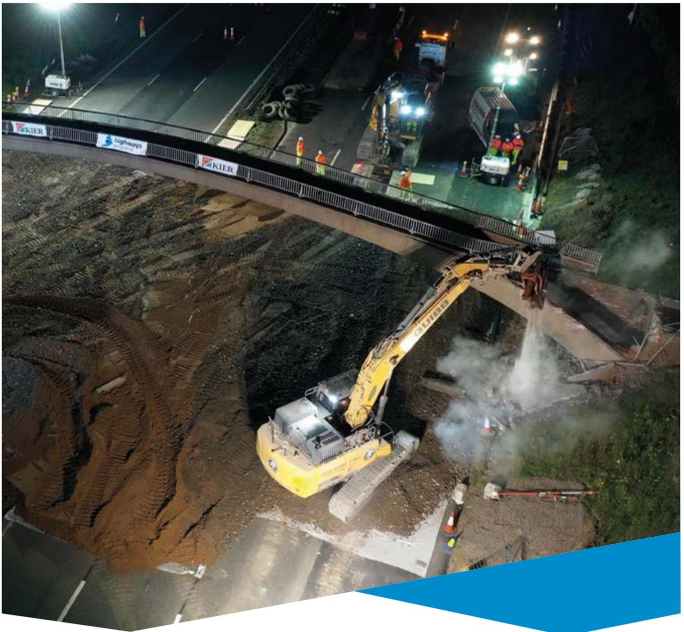
**Picture:** The demolition of Burton Bank footbridge.
