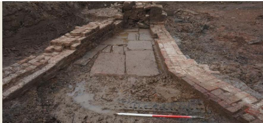
*The headrace channel, with the wooden filter (pierced with holes) in the foreground next to the red and white ranging pole.*
