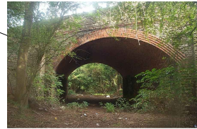
WANSFORD RAILWAY BRIDGE STRUCTURE KEY 7591
