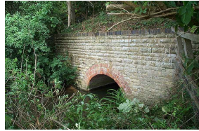
WANSFORD SLUICE STRUCTURE KEY 7590
