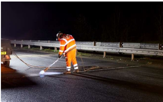
Freshly-laid high friction road surface
