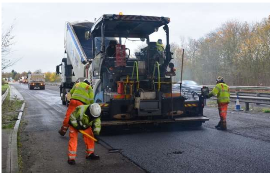
Re-surfacing work underway
