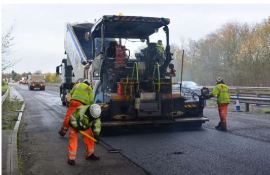
Re-surfacing work underway
