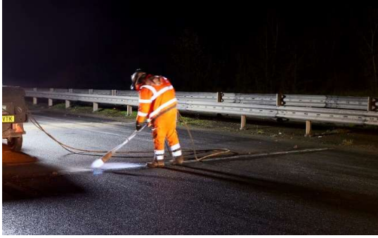
Freshly-laid high friction road surface
