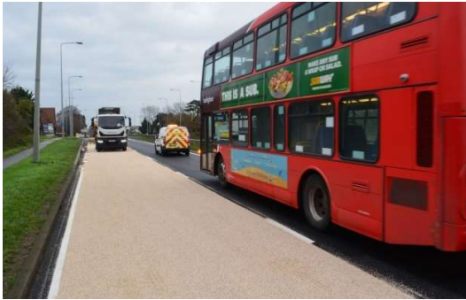
Freshly-laid high friction road surface
