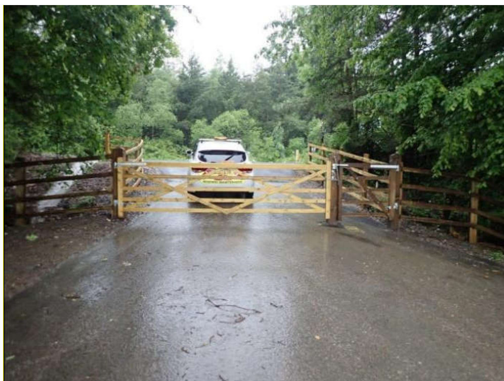
Figure 2-3 Photo gives no context to demonstrate concern described
