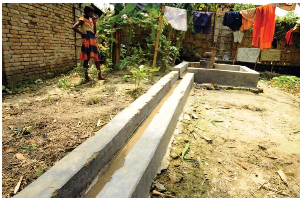
Drainage platforms have helped reduce bacterial contamination and improved the quality of drinking water in Bihar villages
