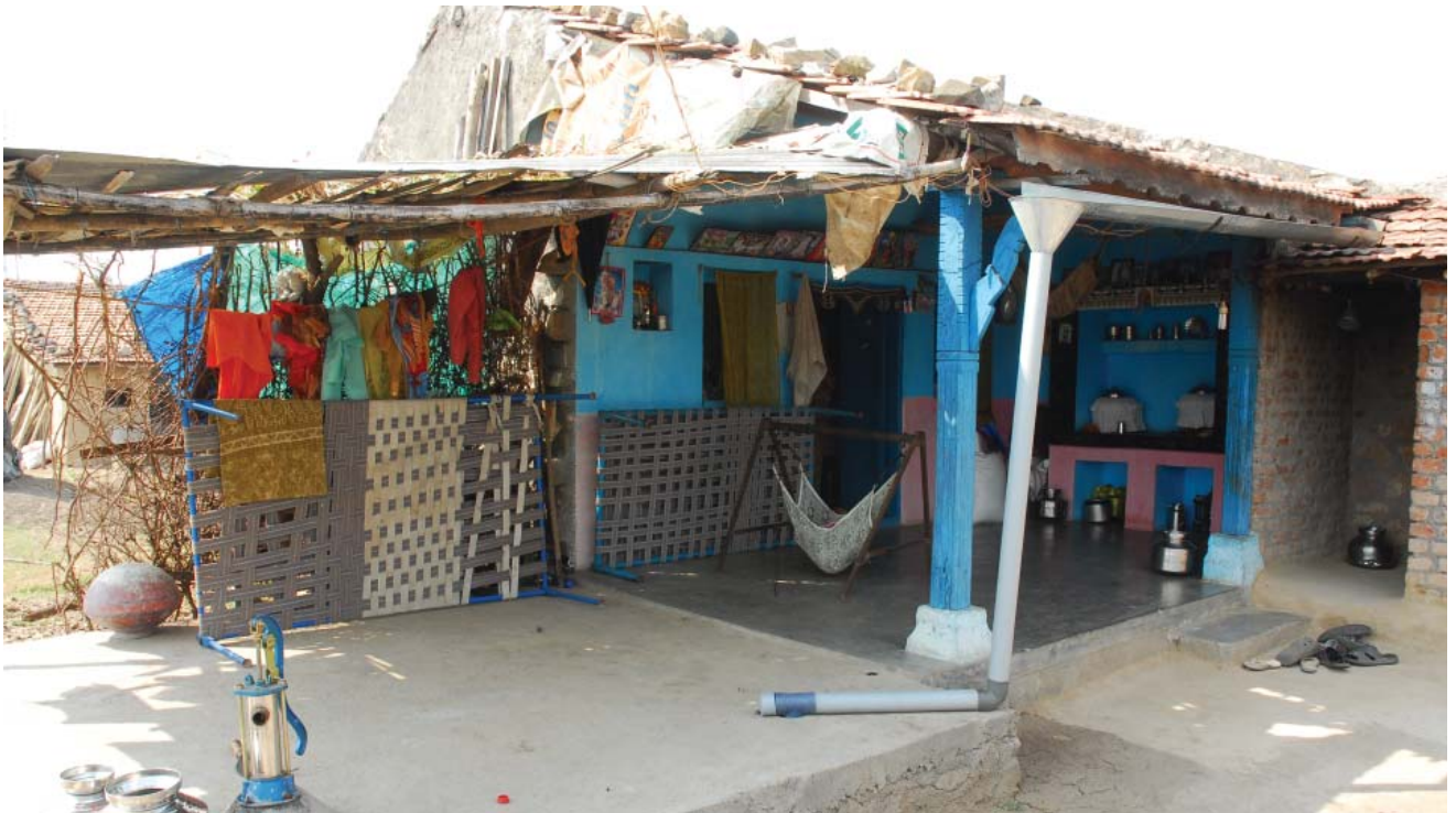
One of the many roof rain water harvesting structures constructed by AKRSP (India) for socially marginalized communities in drought prone Surendrangar
